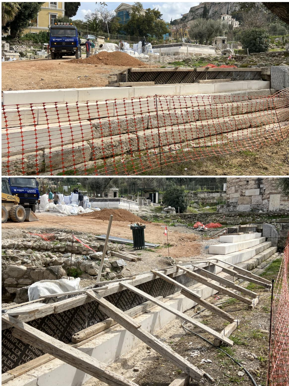
FIG. 9. On top of original Roman steps, before the east end of the Middle Stoa in the Athenian Agora, new steps are being “reconstructed” in reinforced concrete.
