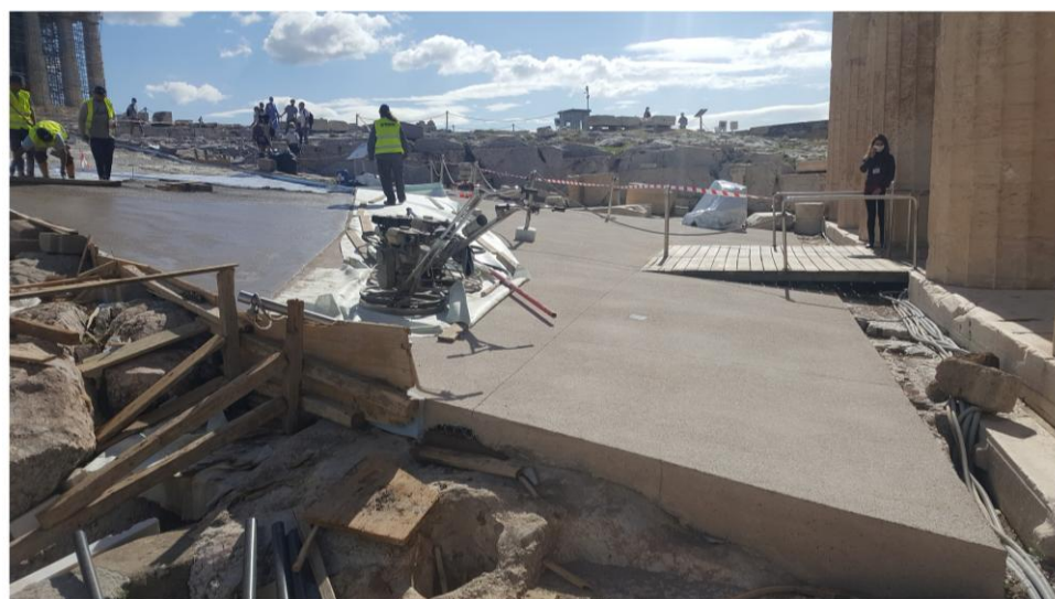
FIG. 1b. The area east of the Propylaia, in the process of being paved with reinforced concrete, covering over the face of the living rock. The wet cement on the picture's left end is covering the plastic sheet and metal mesh, seen in FIG. 1a.
